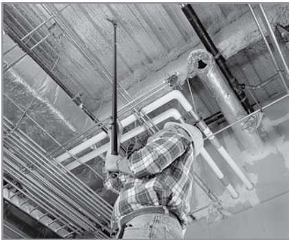
Ramset Pole Tools are an excellent choice for high-reach fastening applications.
