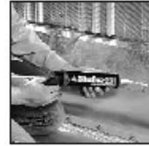
4. Apply additional sealant to both fastened edges for maximum weather-tight sealing.
