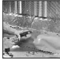
3. Position top edge of Dekstrip over seal bead and install Buildex fasteners at 1-1/2" maximum intervals on top edge. Repeat steps 1, 2, and 3 for the bottom edge.
