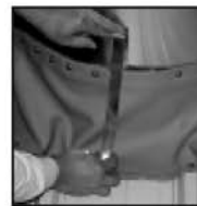
4. Fold termination strip in half, cut to width, and slide over spliced area.
