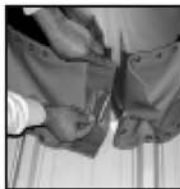
2. Remove film from top of splice tape.
