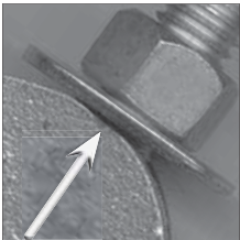
Flat washers provide minimal contact which can weaken the connection and cause loosening of the nut.
